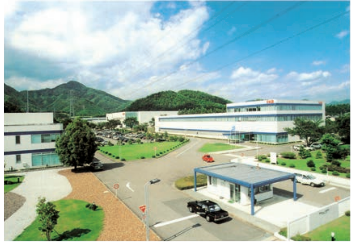
Gifu factory main entrance
